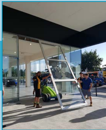
Here is a Winlet 1000 installing some large doors.
