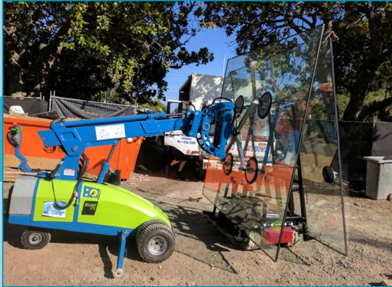
A Winlet 575 loading a double glazed unit onto a Hoeflon Tracked Carrier
